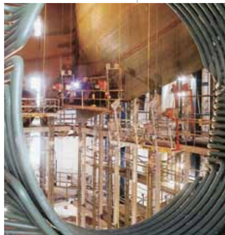
Use of composite tubes in waste incineration plants / biomass fired power plants.
